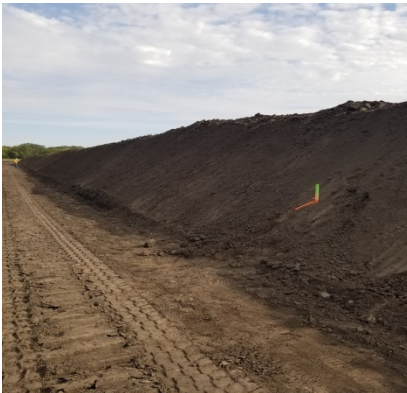
Picture of the dirt piles at SSKP 1042.300 Taken facing North East
